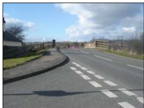
Photograph Four: Visibility to the left from Tatenhill Lane along Branston Road from 2.4 metres set back distance
